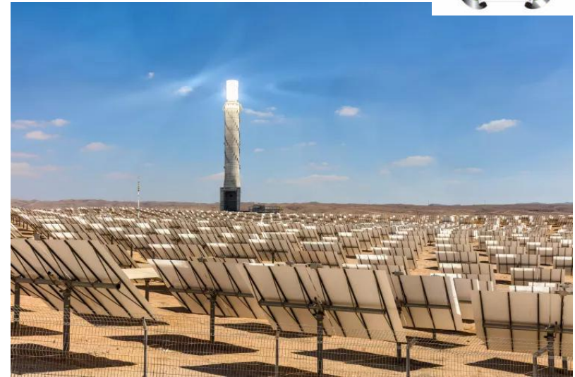
Ashalim Solar Thermal Power Station 121 MW - Be'er Sheva Israel
