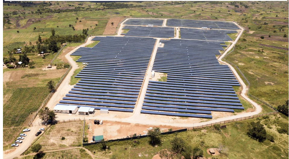
Tororo Solar North Plant, Uganda – 10 MW
