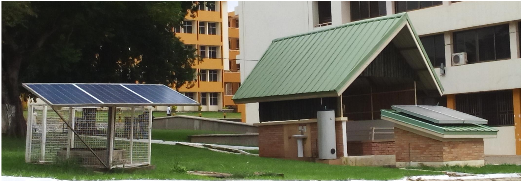
Hybrid solar PV and water heating system installation at KNUST Kumasi Ghana
