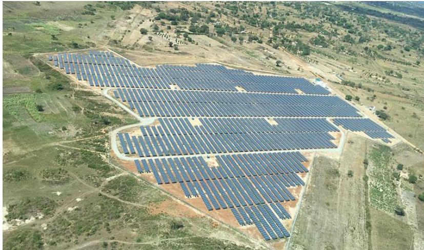
Soroti Solar Power Plant, Uganda – 10 MW
